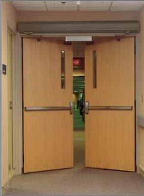
Fire doors are rated to withstand a fire for a specified amount of time. This delays the spread of smoke or fire and gives people extra time to escape.
