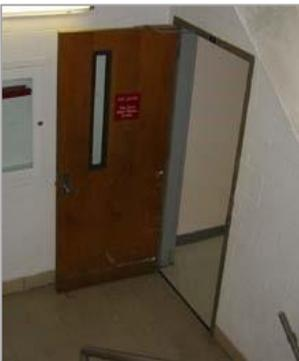
In a fire, stairwells with fire doors propped open to act as chimneys allowing fresh air to reach the fire. An open door allows the smoke and fire to spread to other floors quickly.
