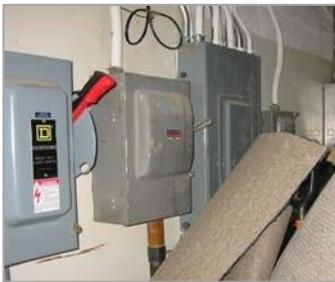
In the event of an emergency, electrical panels must be immediately accessible so that power can be shut off quickly when necessary.
