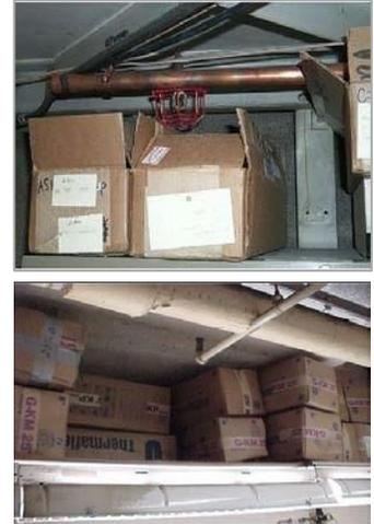
The 18-inches is a continuous plane. You can't build a void around sprinkler heads and expect them to work.
