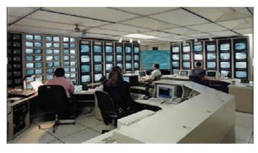
Advanced Traffic Management Systems (ATMS) involve the use of surveillance technologies (e.g. machine vision devices, sensors, and CCTV) and advanced communications (e.g. VMS, HAR, and personal communication devices) to maximize throughput and safety.
