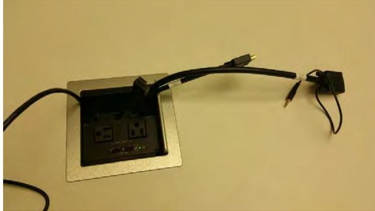
Each VGA cable has been labeled. Plug one of the VGA cables into your laptop's VGA port and take note of the cable's label. Refer to the panel instructions to switch the TV to your laptop's video connection. (If you used the cable labeled "VGA 1" you would press the VGA 1 button on the panel to switch to that particular video source. The image below shows what the VGA cable will look like.
