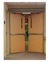
Fire doors are rated to withstand a fire for a specified amount of time. This delays the spread of smoke and/or fire and gives people extra time to escape.
