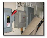
In the event of an emergency, electrical panels must be immediately accessible so that power can be shut of quickly when necessary.
