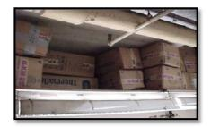
The eighteen inches is a continuous plane. You can't build a void around sprinkler heads and expect them to work. Call the Warehouse. Call the Hazardous Materials Facility for pickup. Call somebody to clean this mess up!
