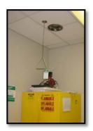
This shower was originally installed in this ceiling for a reason. Nothing should obstruct a person's access to it.
