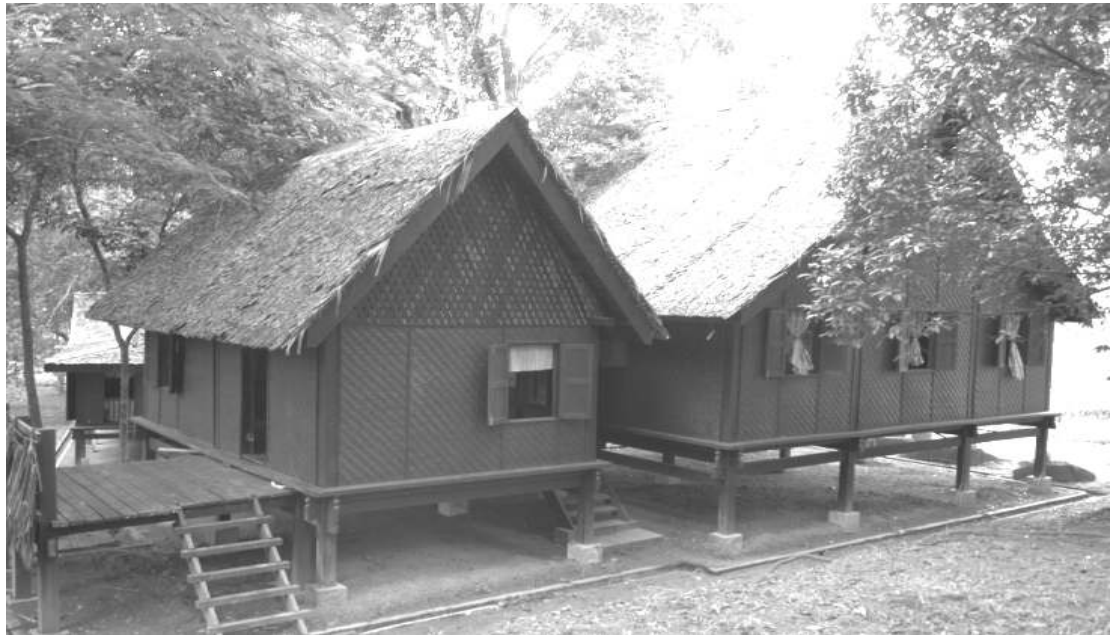
Figure 3: A traditional Malay house showing a main house, a kitchen annex and a washing place.
