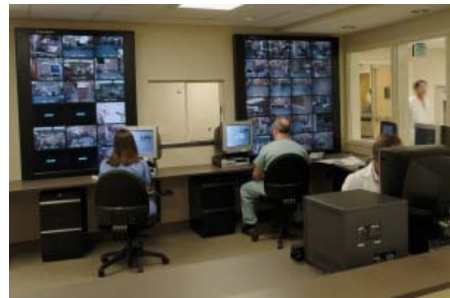
Video-screen control boards let staff keep an eye on all of the operating suites on each floor at a glance.
